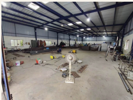
Fabrication shed Steel-framed, open span.
